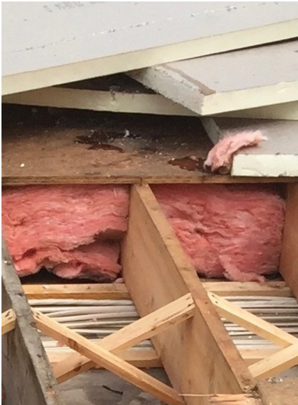
10" fiberglass plus 4" ISO board – R50 total.
