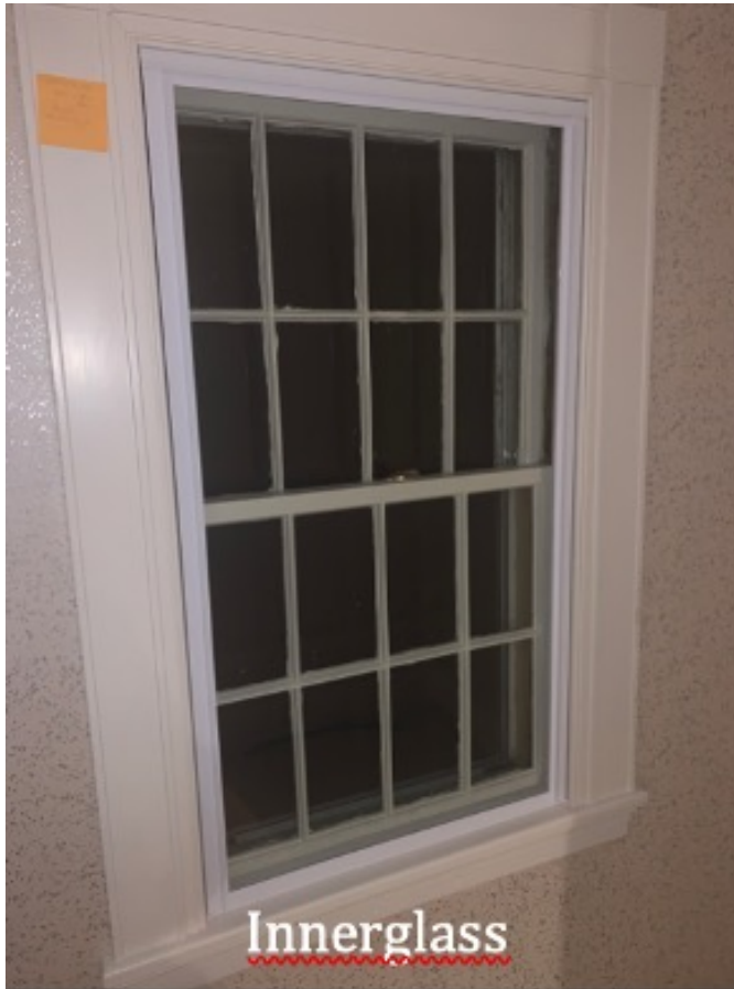
Window insert in single-pane window.
